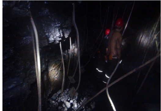
锚杆弯曲悬吊
